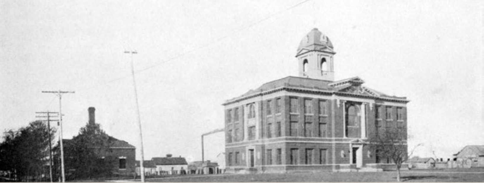
ABOVE Cleveland County Court House, c. 1906. This was later demolished by WPA workers. Norman, OK Collection, no. 8
